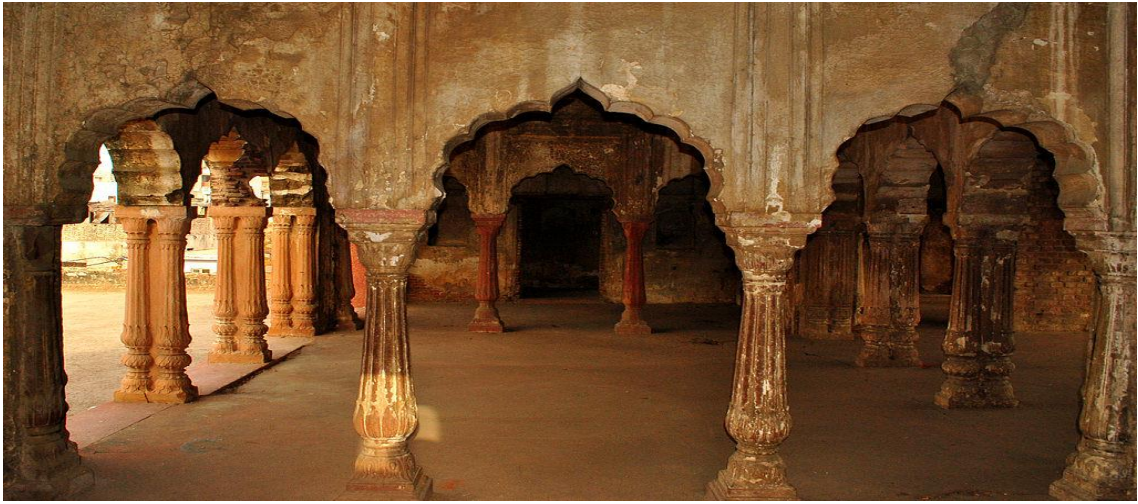
Upper Storey of the Gate.
