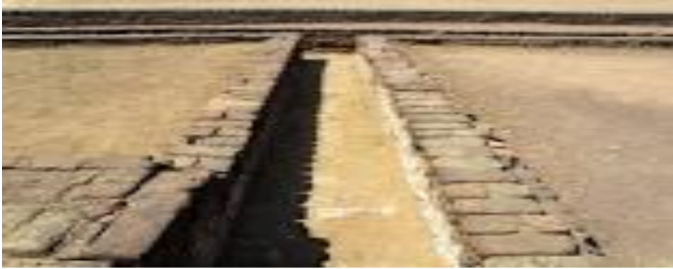
Drainage in Lothal
